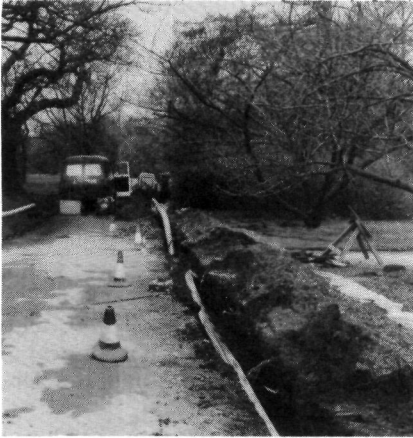
Left: Laying gas main near King William's Temple.
