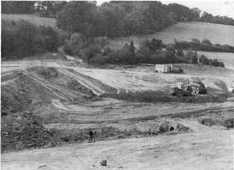
The new reservoir at Wakehurst Place under construction.
