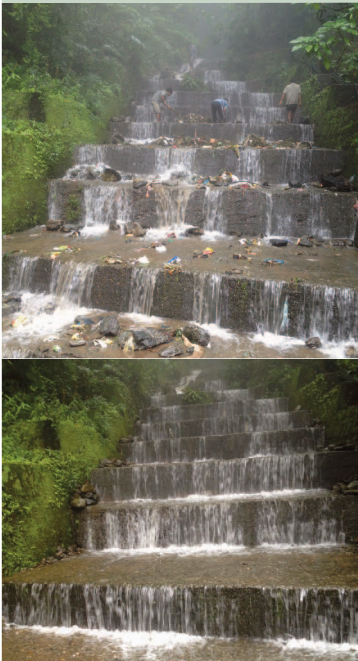
The rivulet, before and after cleaning
