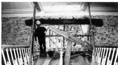
Work in progress inside Museum No. 1.
