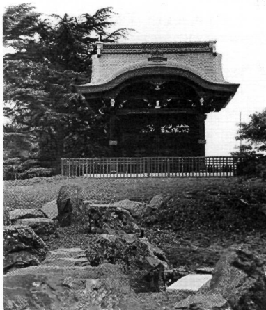
The Japanese Gateway – the new landscape surrounding the restored Gateway being constructed by Japanese craftsmen alongside Kew's Arboretum staff.
