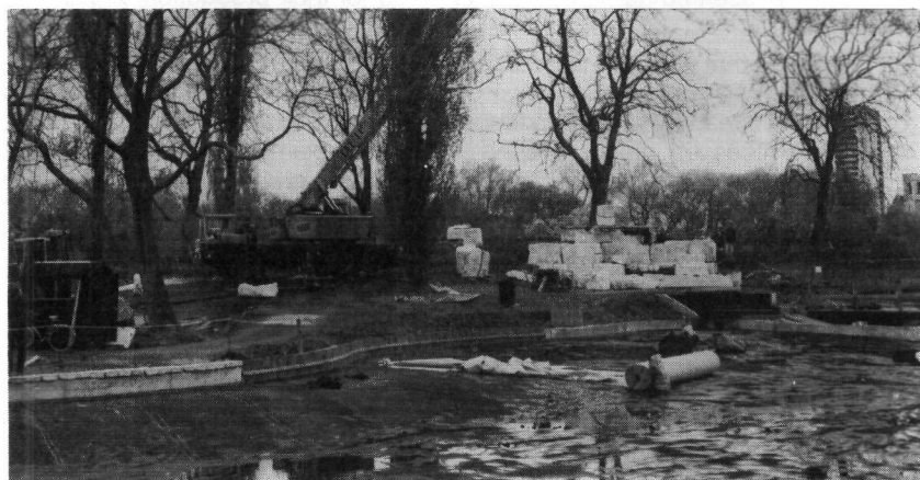
Cascade construction. Upper lake with butyl liner in place.
