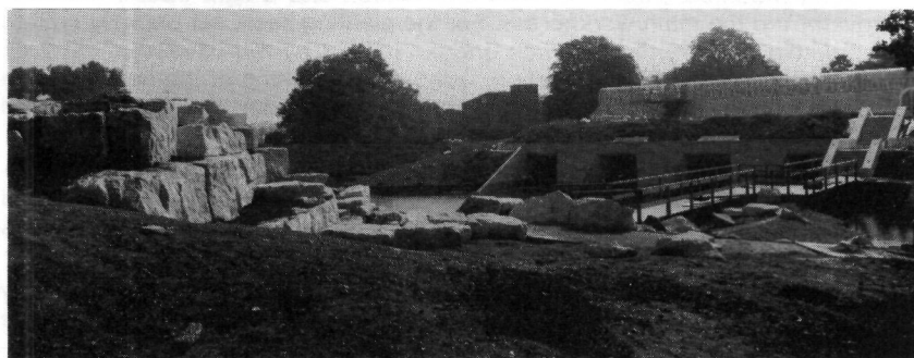
Cascade, boardwalk and roof garden under construction.
